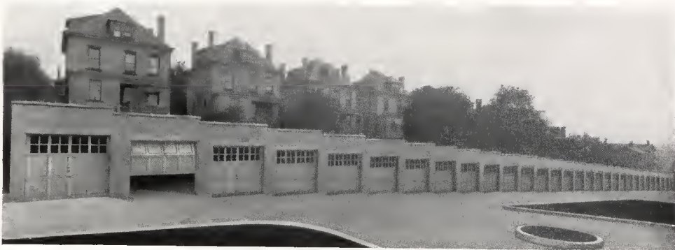
An installation of thirty No. 900 Door Sets at Bellevue, Pa.
